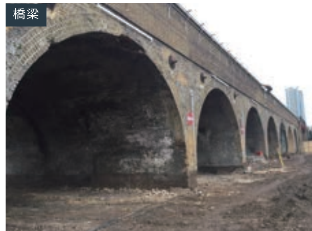
Masonry Arch Bridge, Roma-Formia railway line in Italy
